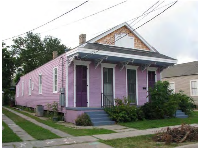
Photograph 1. 439-41 Angela Avenue, Old Arabi Historic District (April 26, 2009).
