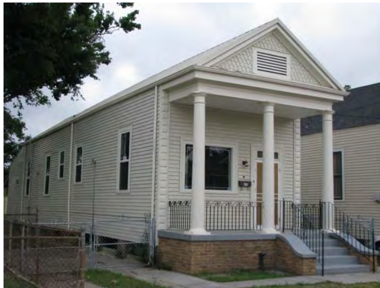
Photograph 1. 635 Angela Avenue, Old Arabi Historic District (April 26, 2009).
