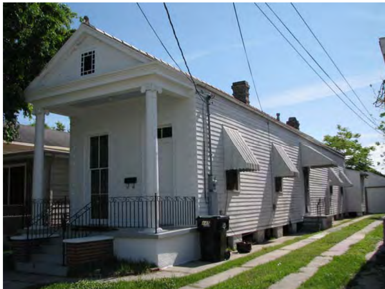
Photograph 1. 445 Angela Avenue, Old Arabi Historic District (March 30, 2009).
