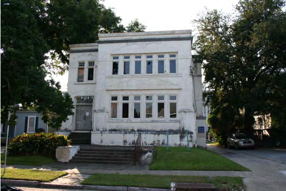
Figure 2. Main Façade, 1021 Audubon Street.
