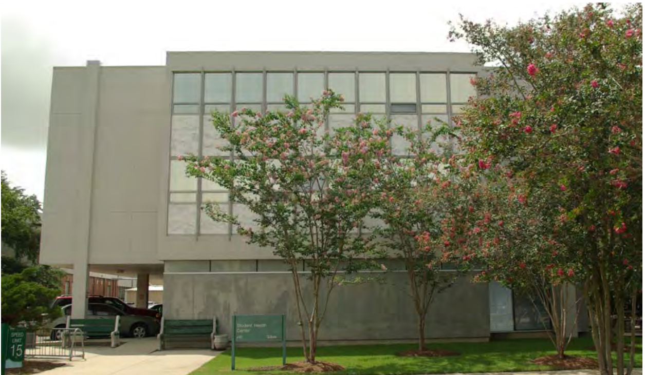
Figure 10: Building 84: Caroline Richardson Building
