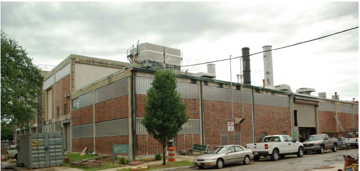
Figure 7: Building 86, Power Plant Building
