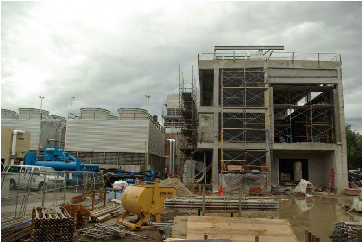
Figure 9: Building 92, Student Health Center
