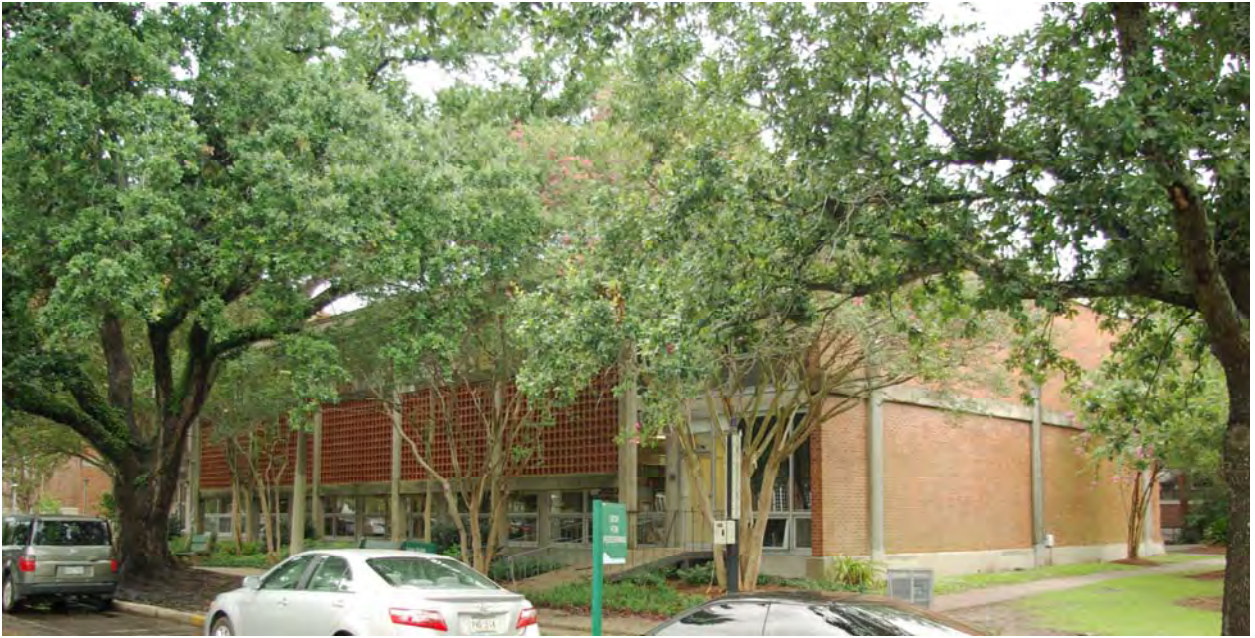
Figure 11: Building 85, Physical Plant Building
