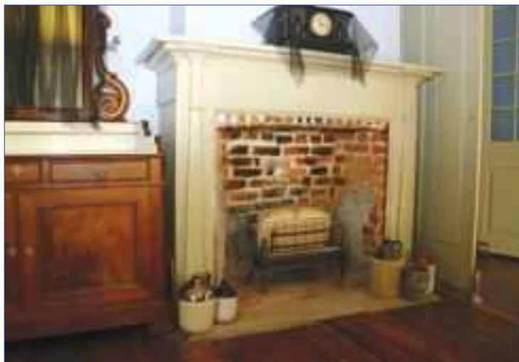
Restored firebox and French wraparound mantel at Sebastopol.
