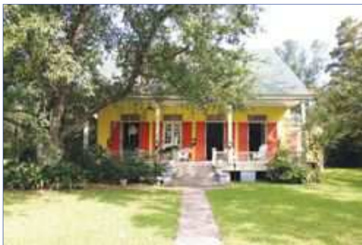
Sebastopol's restored porch and façade.
