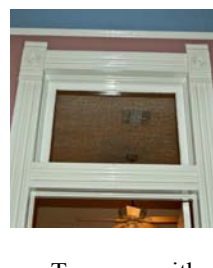
Transom with Decorative Surround
