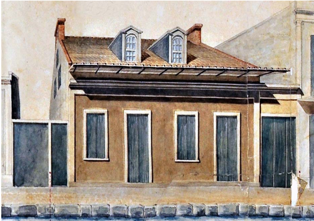
Fig. 5.39a. The Arsène Latour atelier, 625-627 Dauphine Street, dating from 1808 - 1813. This is a platibanda cottage with a cymantia cornice and an unusual asymmetrical façade. A sleeping loft has been added under the steeply pitched roof. The chimneys are lower than on cottages of the first decade. The color scheme is among the most popular on Creole cottages 1804 – 1825. The image has been modified in Photoshop to conform to the geometry of the surviving facade.
