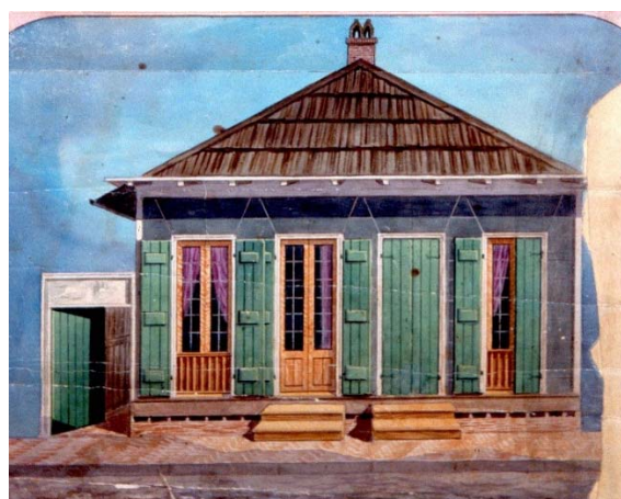
Figs. 5.27 and 5.28. Examples of two forms of early linear cottage, both covered with merrains . The single wide cottage on the left was built by Pierre Roup, a Saint-Domingue refugee and builder who arrived in New Orleans ca. 1805. This house was located at 1744 N. Rampart Street, and is no longer standing (NONA 089.024). The cottage on the right is the ca. 1810 Phillipon Cottage, which still stands on Dauphine Street in a somewhat changed appearance (NONA 044.035).
