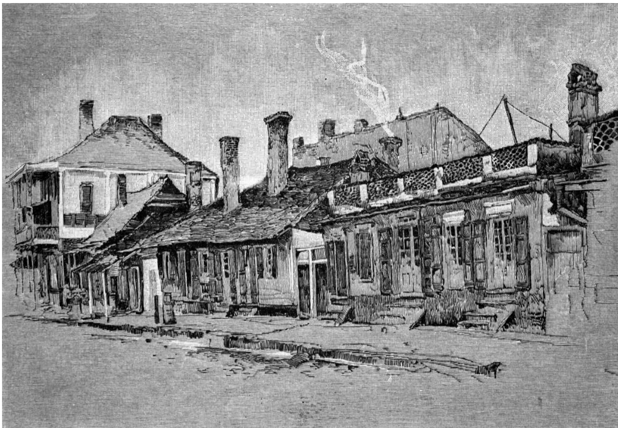
Fig. 5.20. Two terrace-roofed cottages at 707-709 and 711- Dumaine Street (far right side of image). These were probably designed and built by Barthelemy Lafon in 1799. The cottage at the far right, the de la Torre house, survives. The cottage in the left-middle of the image also originally had a terrace roof which was covered over with a pitched roof at some later time, probably in the first decade of the 19 th century. Sketch by Joseph Pennell.
