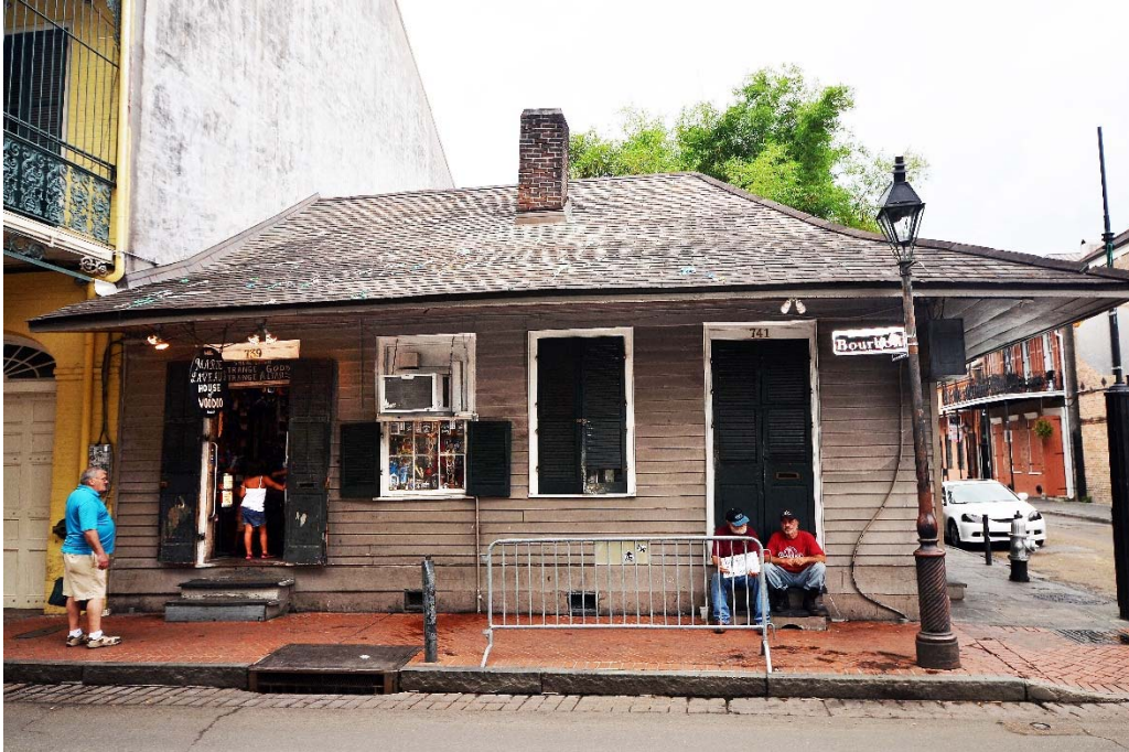
Fig. 5.32. 739-741 Bourbon, a half-hip, half-gabled roof corner cottage at the intersection of Bourbon and St. Ann Streets. 739 Bourbon Street functions as a corner store. The abat vent wraps around the corner. Many other corner cottages have a similar configuration JDE Photo 2014.
