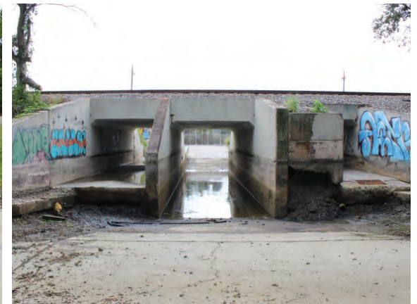
Entrance Tunnel, facing southeast, remaining
