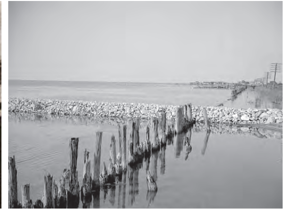
Breakwater Structure, remaining
