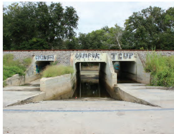
Entrance Tunnel, facing northwest, remaining
