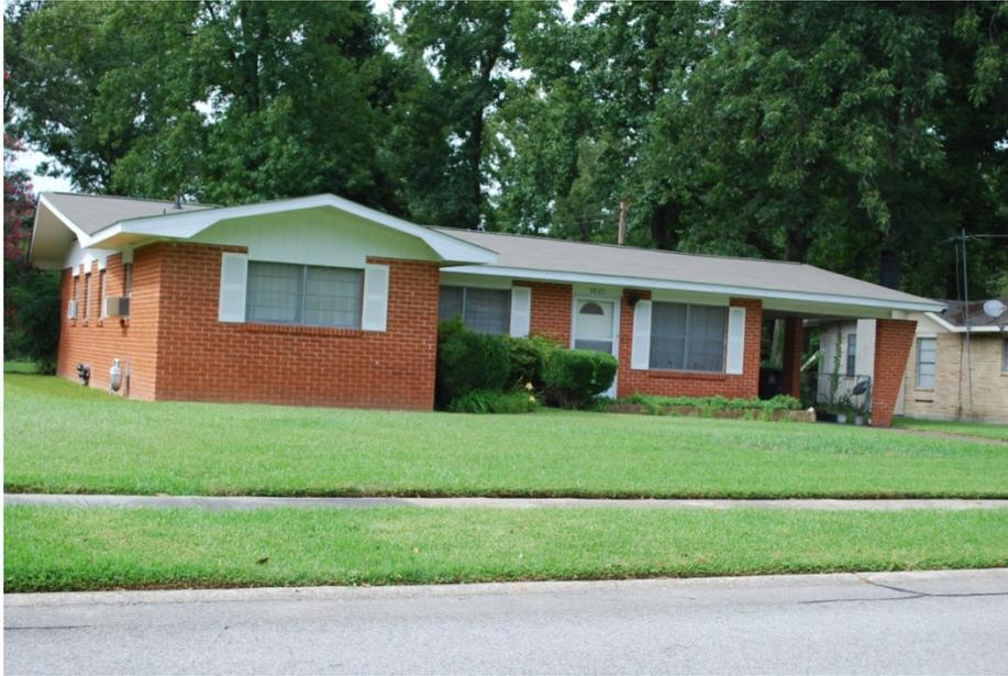
**Photo 1. This Baton Rouge ranch house illustrates several character-defining ranch house features: one story with a low spreading horizontal emphasis; long side parallel to the street; low pitch roof with moderate to wide overhanging eaves.**
