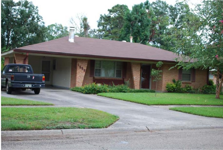
**Photo 5. Note the picture window with flanking four pane windows.**
