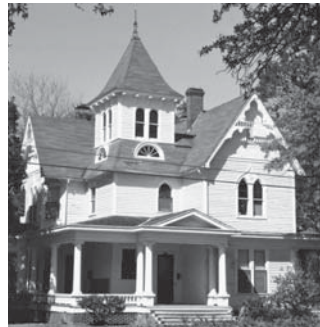
The tower on this Lake Charles Victorian residence is an important part of its design. Were it to be lost, the home’s National Register design integrity would be severely compromised.
