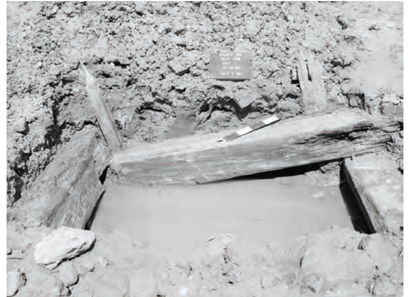
(Top) Closeup view of sandstone boulder concentration in crib section of Lower Bailey's Dam, facing north. Courtesy of the Library of Congress: HAER LA, 40-ALEX. V,2-17.
