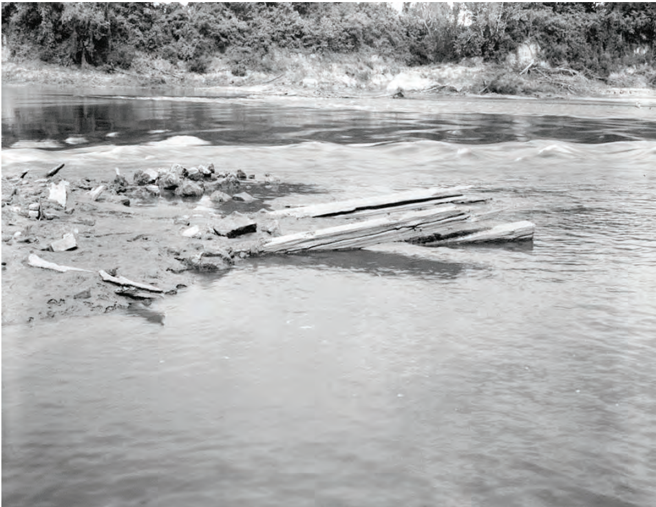
(Above) Closeup view of exposed crib timbers from crib section of Lower Bailey's Dam, facing northeast. Courtesy of the Library of Congress: HAER LA, 40-ALEX. V,2-16.
