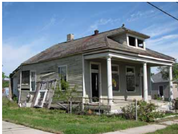
Photograph 1. 750 Angela Avenue, Old Arabi Historic District (March 30, 2009).
