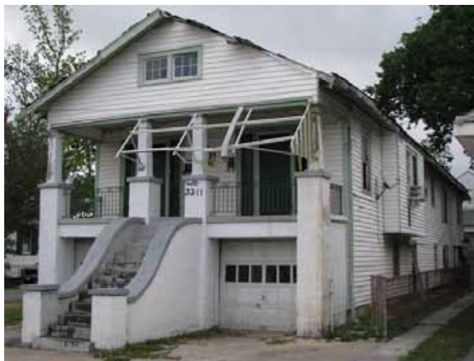
Photograph 1. 647-49 Angela Avenue, Old Arabi Historic District (April 27, 2009).
