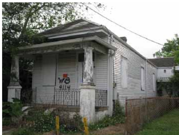
Photograph 1. 523 Angela Avenue, Old Arabi Historic District (April 27, 2009).
